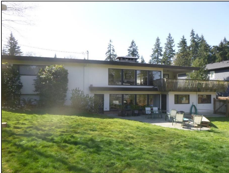
Plate 2. View of north side of subject property, looking approximately south.
